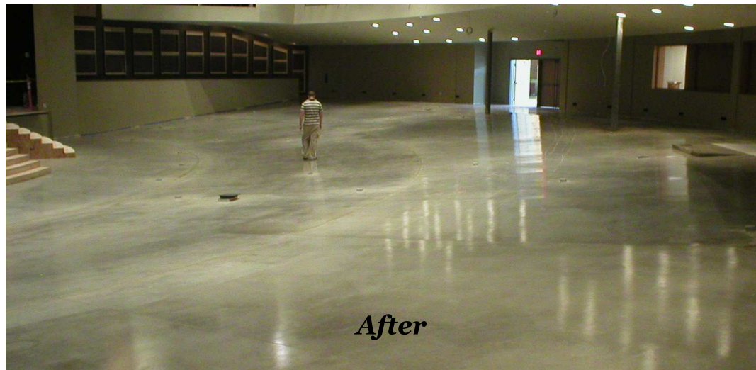
Church - Lisle, IL The HP-105 Clear was applied to bare concrete.
