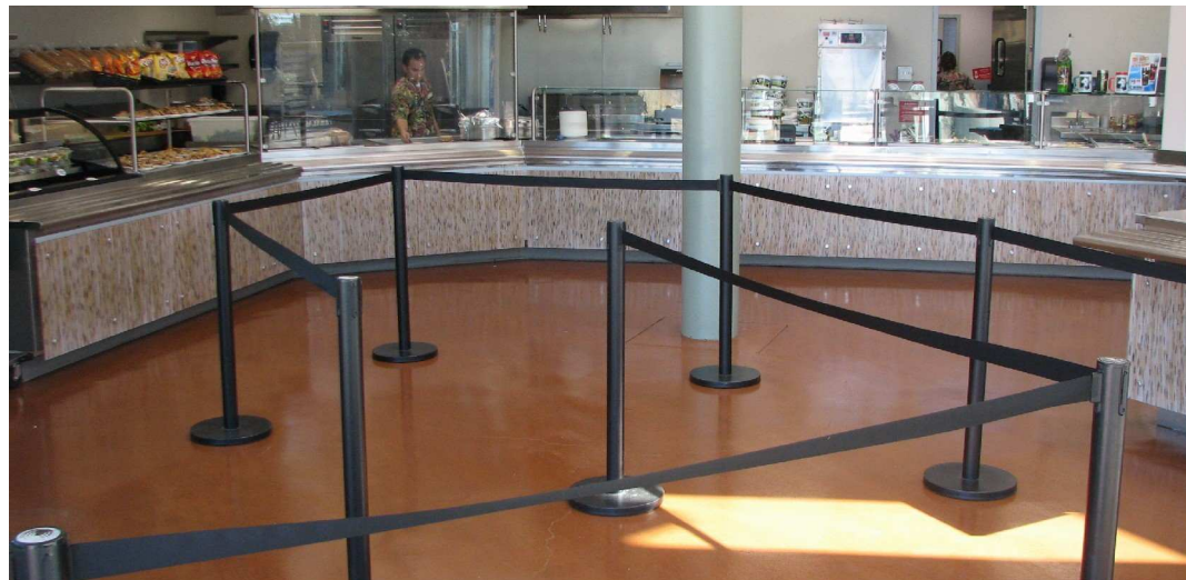
San Diego Zoo - San Diego, CA The HP-105 Clear was applied over a stain on concrete in the cafeteria and gift shop.
