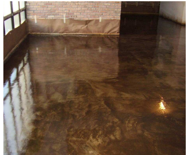
Refinery Restaurant - Chicago, Illinois The HP-105 Clear was applied to a stained concrete floor.
