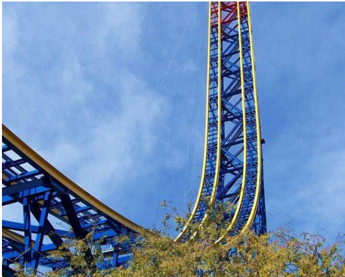
Superman Roller Coaster - Six Flags Magic Mountain - California The HP-105 Blue was applied to the structural steel.
