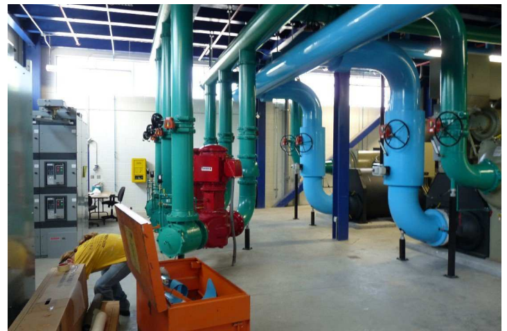
Various HP-105 colors applied to structural steel and piping.
