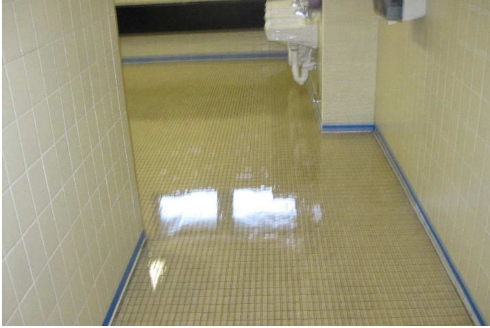
Step 1: Apply the HP-330 on top of the Ceramic to even out the floor.
