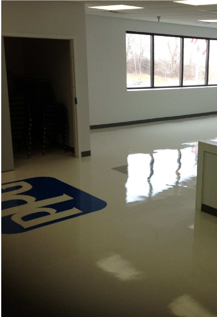
PPG Distribution Center - Batavia, IL The GlossTek Fast Dry was applied to VCT floors of the distribution center.
