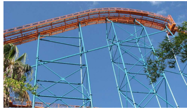
Goliath Roller Coaster - Six Flags Magic Mountain - California The HP-105 Blue & Orange applied to the structural steel.
