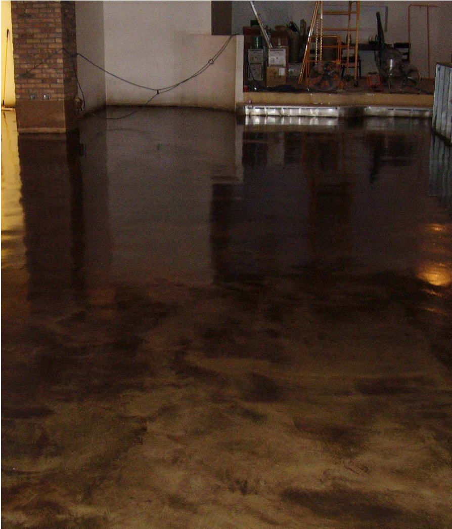
Refinery Restaurant - Chicago, Illinois The HP-105 Clear was applied to a stained concrete floor.
